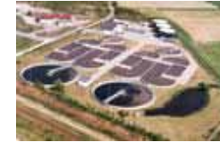
South West Wastewater Treatment Plant (SWWTP) in St. Petersburg (2002)
