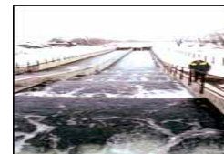
Water Purification Plant in South Butovo (Moscow, 1997)
