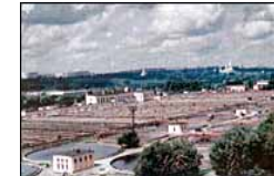
South West Water Purification Plant in Moscow (2004)
