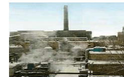
Waste Incineration Plant No.3 in Moscow (2005)
