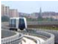
Machinery & Steel Structures
