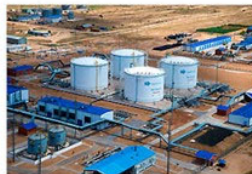
HOPS Kenkiyak Total area 40,000 sq m 148 sensors were installed
