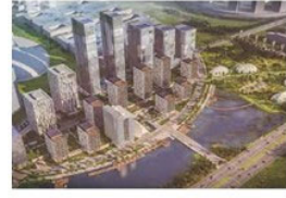
«GREEN Quarter» Total area 75,000 sq m 128 sensors were installed
