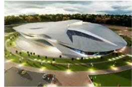
Indoor Pool in Taldy-Qorgan Total area 27,000 sq m 148 sensors were installed
