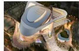
Jekpe-Jek Palace Total area 75,000 sq m 188 sensors were installed
